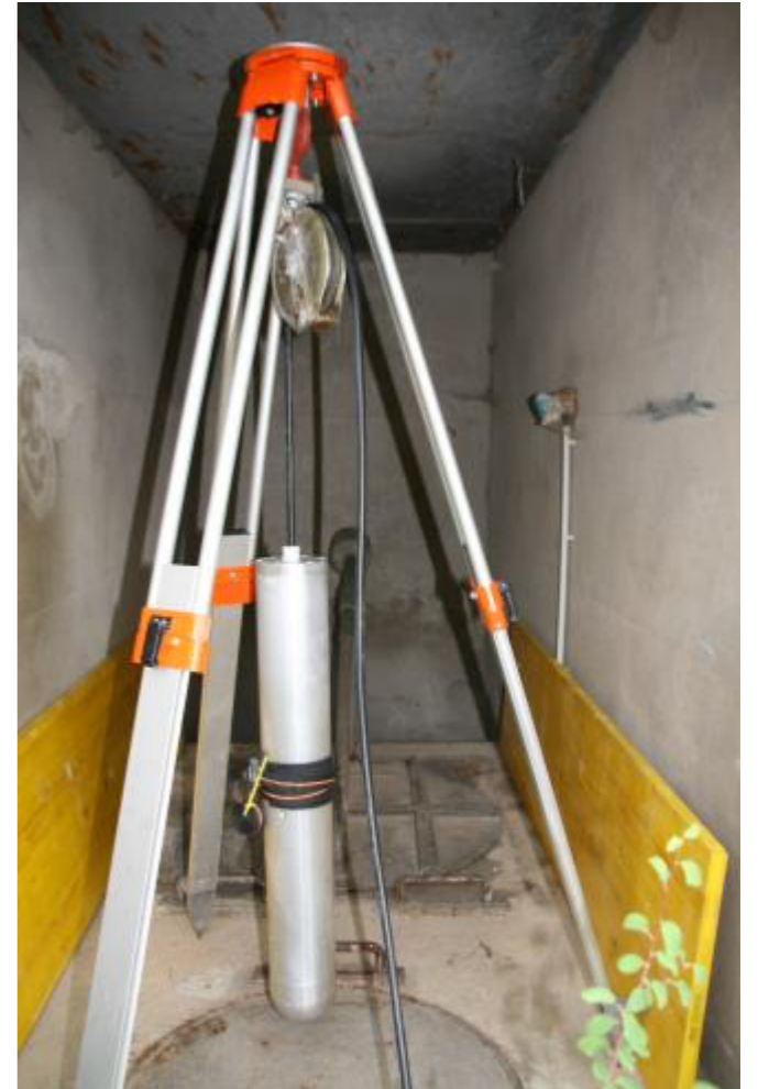
Testing one of the downhole tools
