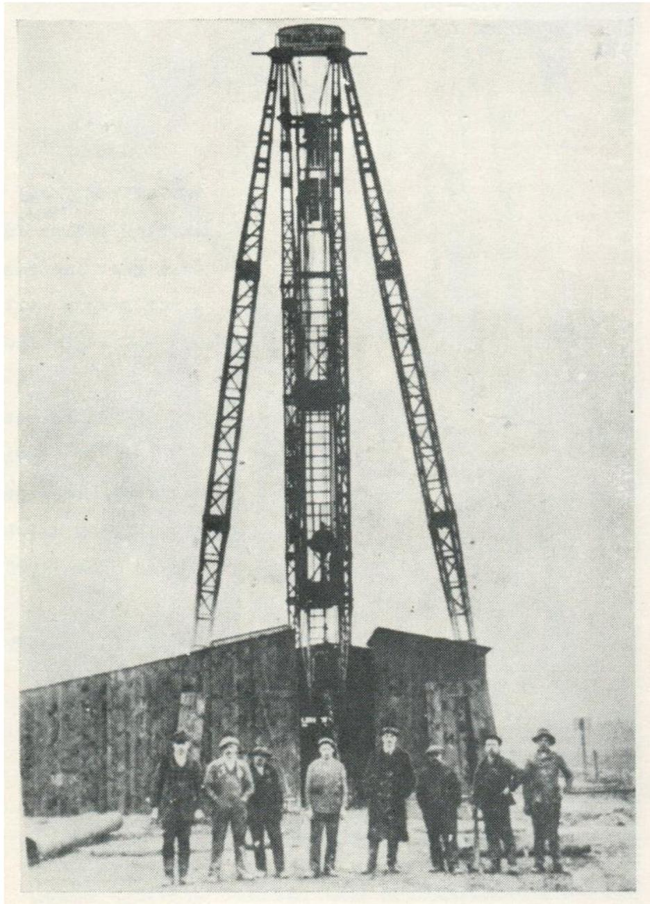
Figure 11. Drilling rig Trauzl-Rapid and oil rig crew from 1913 – 1914. First production well in the Vienna Basin: Gbely – Old Field – Slovakia (Bednaříková and Thon 1984).
